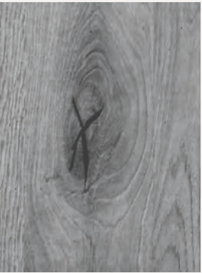
FK / FILLED KNOTS The knots are filled and the wood is planned and sanded to achieve a smooth surface.
